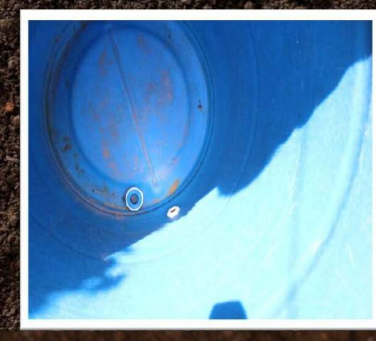
Once the opening is made, the tap is inserted and then attached inside via a plastic nut. A pliers may be used to tighten the nut.
