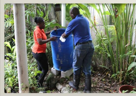
You can add another pipe to the house's gutter system to channel rainwater into the drum.
